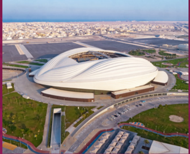
Al Janoub Stadium
